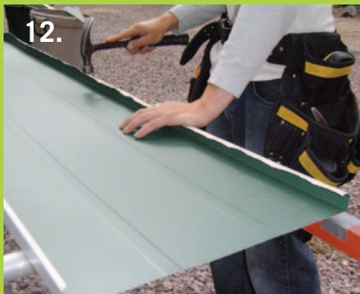
11 & 12: Fabricating a double male panel from a standard roofing panel.
