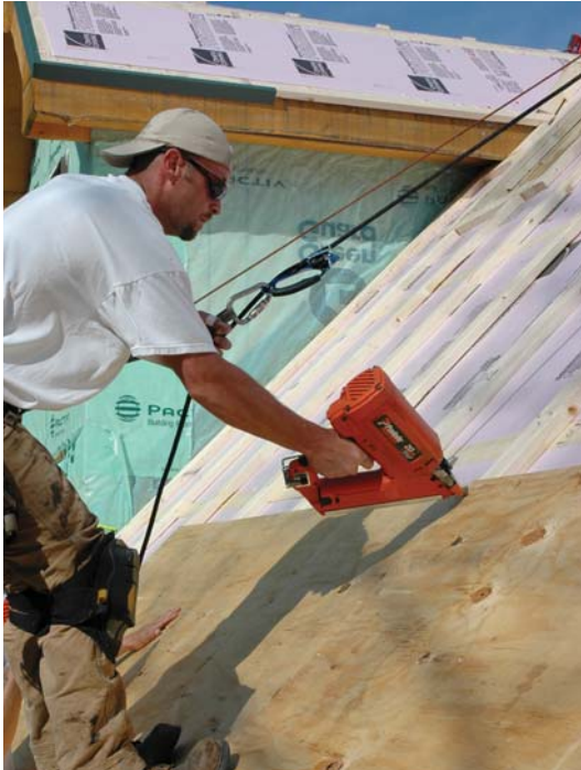
Figure 3. The roof sheathing is fastened to the 2x4 spacers, creating a 1½-inch vent channel above the rigid foam insulation (left). The sheathing stops short of the peak to allow airflow through the ridge vent (above).
