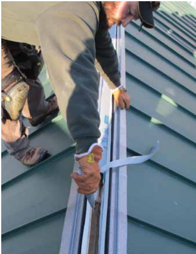
Left: Underlayment is removed to expose venting just before cap is installed.
