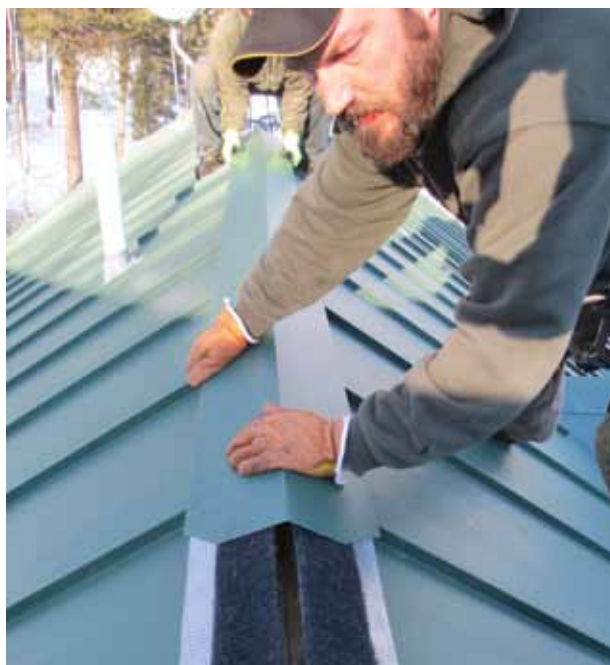
Ridge cap is applied by sliding it onto the vent assembly.
