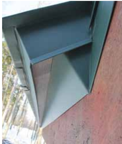
Eave venting applied over existing roof deck.
