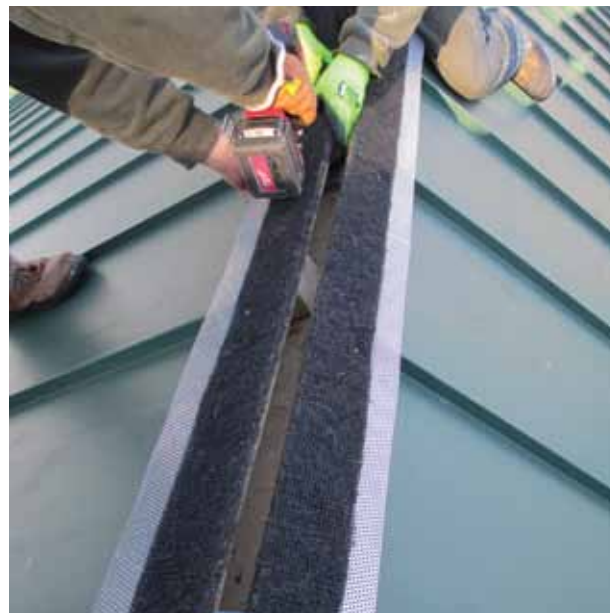
Below: Venting fabric is applied into ridge with zip screws to prevent fine snow from infiltrating.
