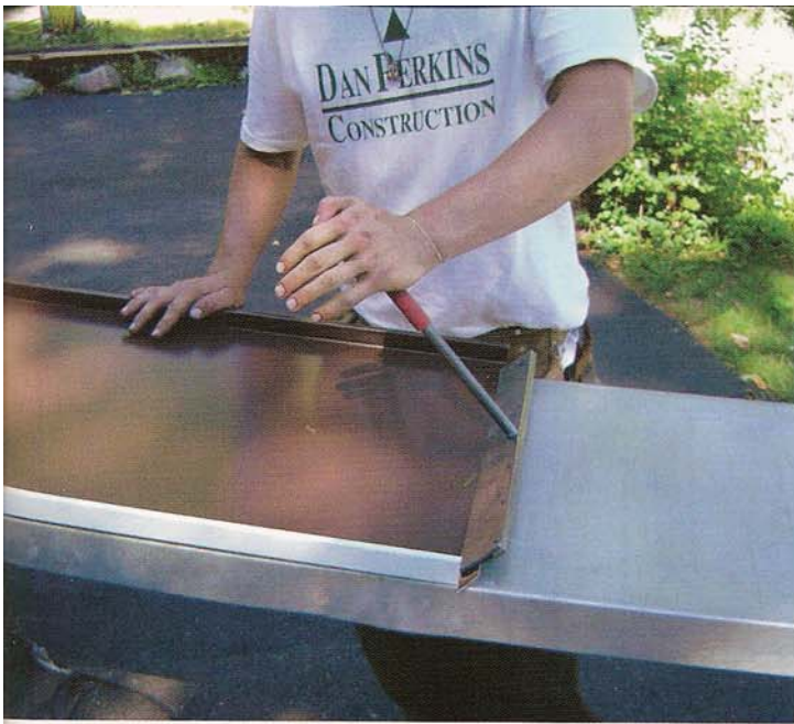
The roofing pans are "box panned" before they are installed into the ridge, and baffles are applied to prevent wind from driving water and snow directly into the perforations in the C channels.
