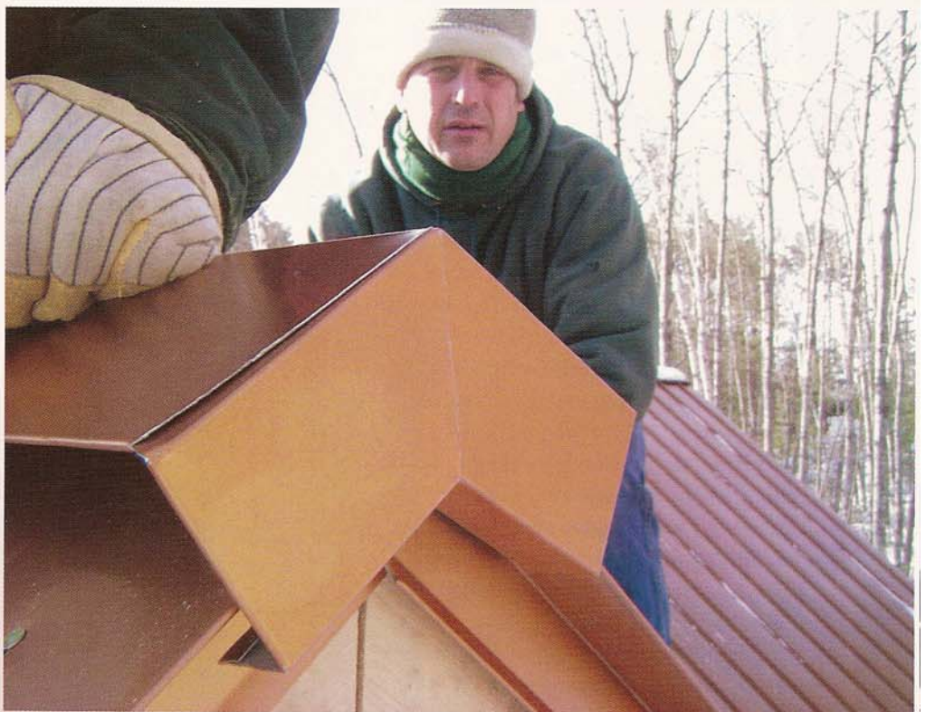
The ends of the ridge are closed with an end cap that is slid into the hem holding the cap to the perforated C channels.
