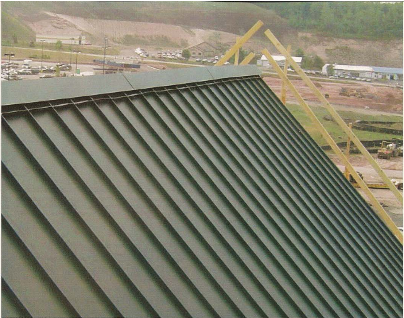
The ridge vent and cap shown are designed to be installed before the roofing panels are installed. This has proved to be a watertight system that can be applied more efficiently and safely than ridge caps that are installed after panel installation. Photos courtesy of Dan Perkins Construction Inc., Ishpeming, Mich.
