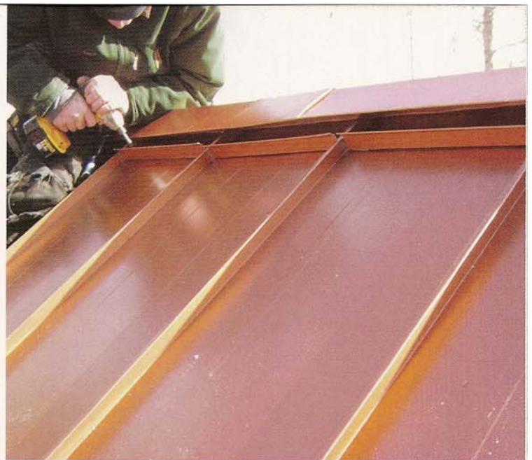
As the wind is diverted around the baffles and over the ridge cap, negative air pressure is created, increasing the air flow out of the roof system. The baffles are applied to the roof panels on a 1-inch (25-mm) butyl tape and screwed down with gasketed fasteners. It is important to leave a gap at the sides of the baffles for water to drain from the ridge assembly.
