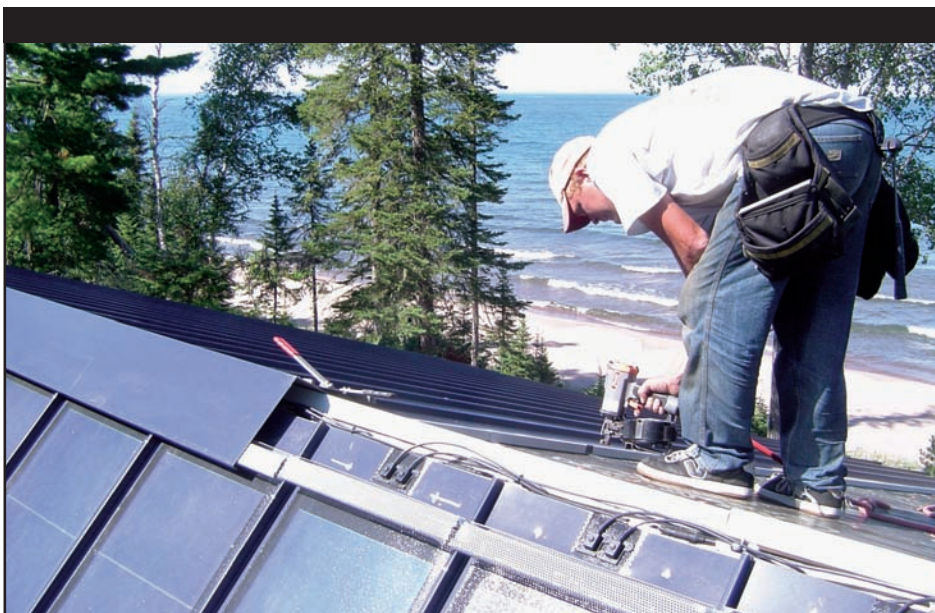
Dan Perkins developed this vented accessible ridge cap to work as a wiring channel for an amorphous film array.
