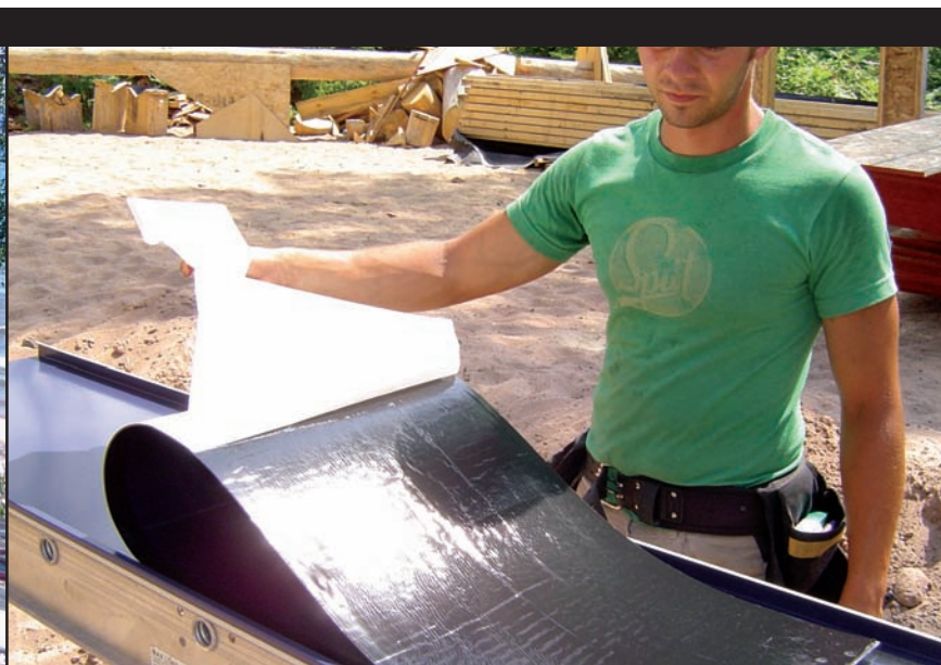
Application of thin film to steel
