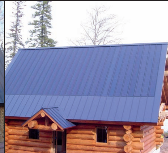
This is a 4-kilowatt, off-grid, amorphous thin film application on steel.
