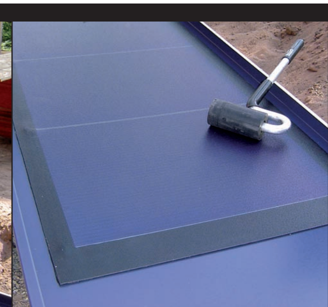
Application of thin film to steel
