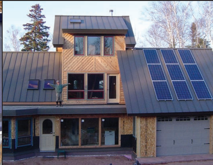
Crystalline modules on a small residence
